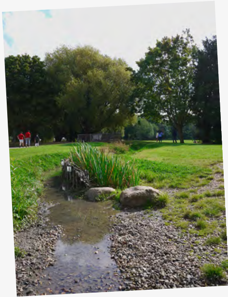
The de-culverted Yeading Brook, Headstone Manor Park
