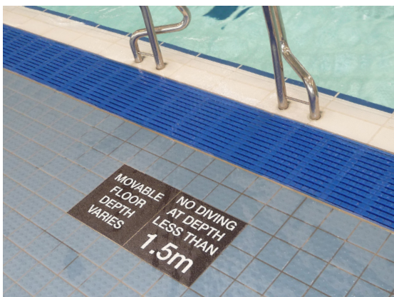
Variable depth (movable floor) marked on the pool surround
