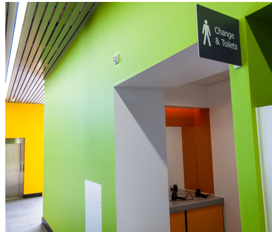
Wayfinding enhanced by the use of contrasting wall colours
