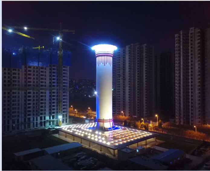
Figure B A night-view of the 1 st generation SALSCS built in Xi'an, Shaanxi Province (completed July 2016)
