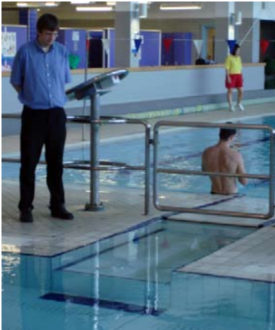
Submersible platform lift at Craven Pool, Skipton
