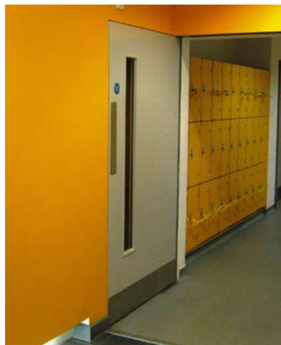
Where doors must swing out into a corridor they should be set in a recess
